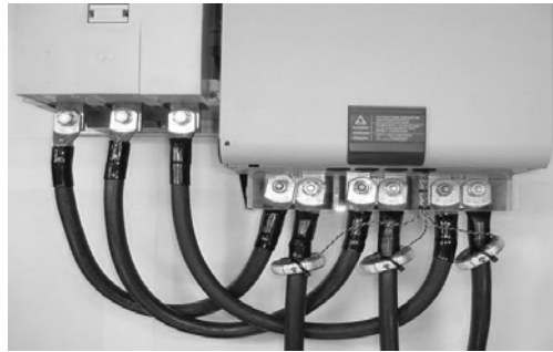
Figure 9.15 - CTs to external current acquisition
