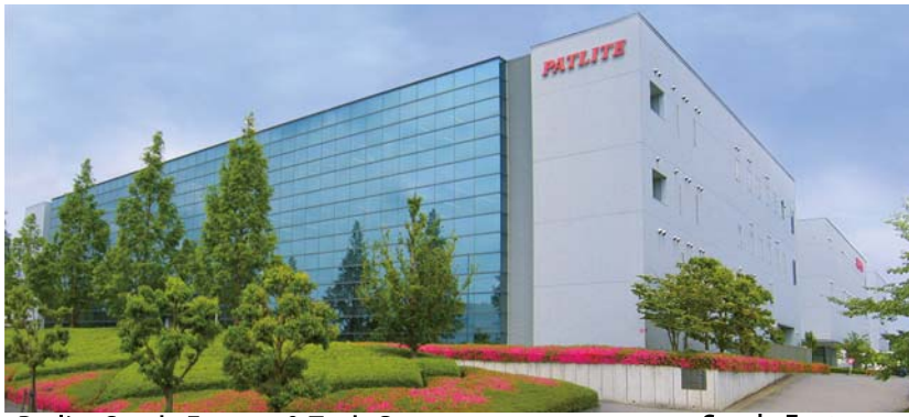
Patlite Sanda Factory & Tech Center
