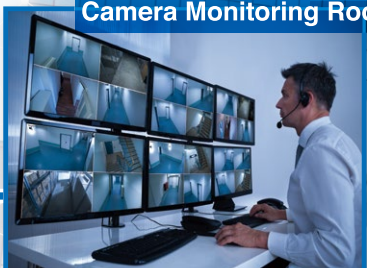
Camera Monitoring Room
