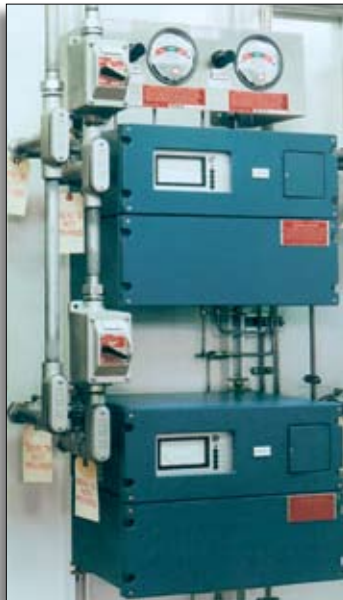
In this application, a dual pressurization system is mounted above two identical devices that are separately protected to allow independent access. Both devices feature TYPE 4 cases, which makes them suitable for purging as is.
